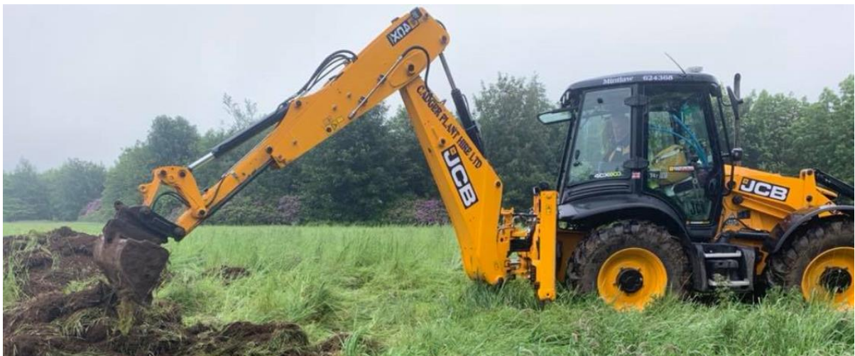
Experience digger driver Robbie Cadger busy at work
