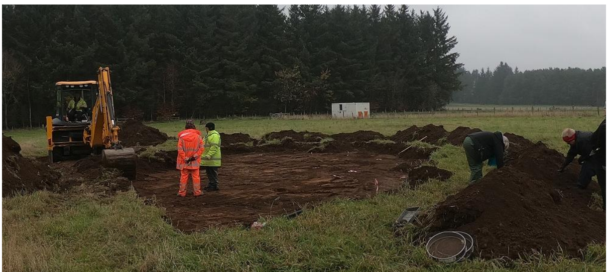
Centre of structure cleared
