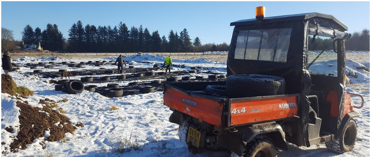
Additional weights/tyres being added
