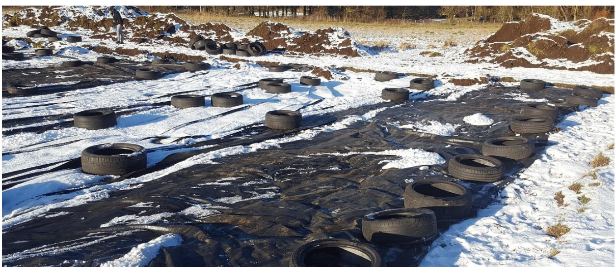
Matting and weight/tyres in situ
