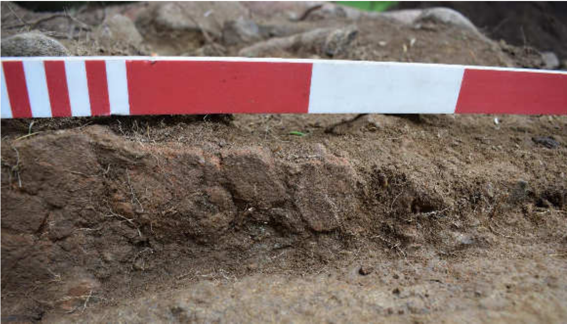
Illus 12 'Plaster' 149 on internal (south) face of N wall 151
