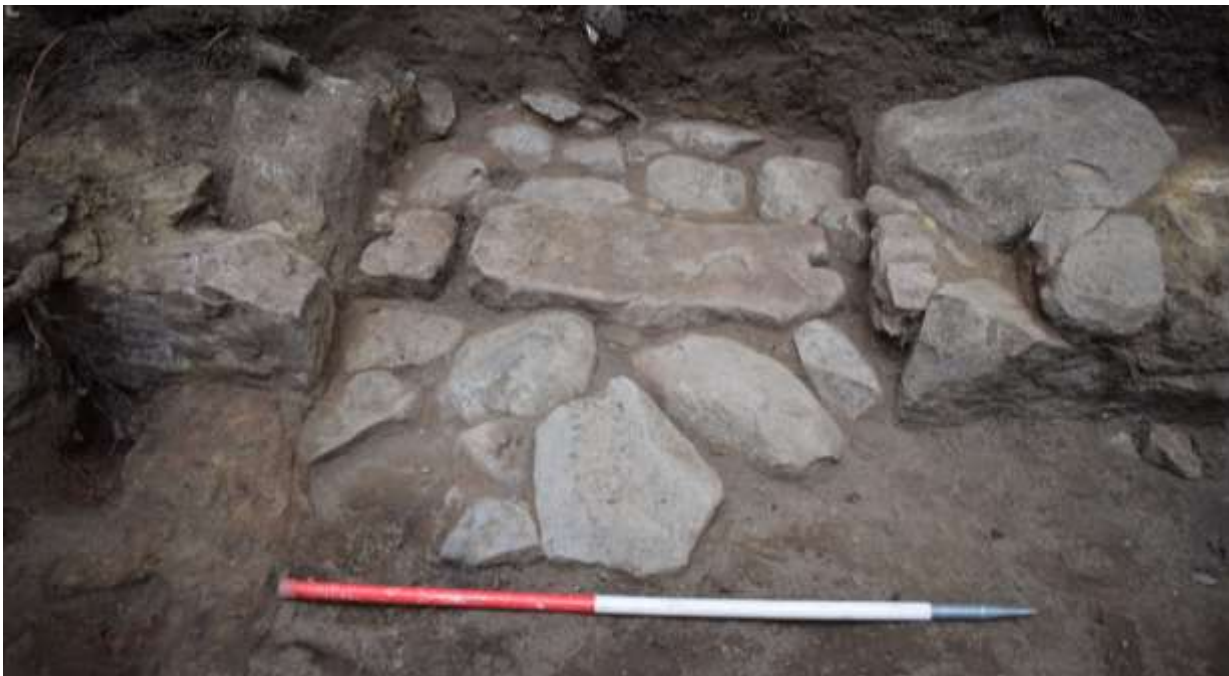
Illus 10 Door 228 with interior cobbles (230; foreground) and exterior cobbles (229, entre top); facing S
