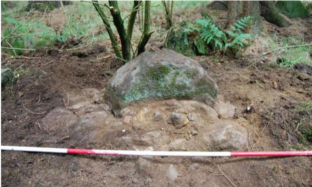
Illus 35 S wall foundation with large curved stone left and reused in Phase 3; facing S
