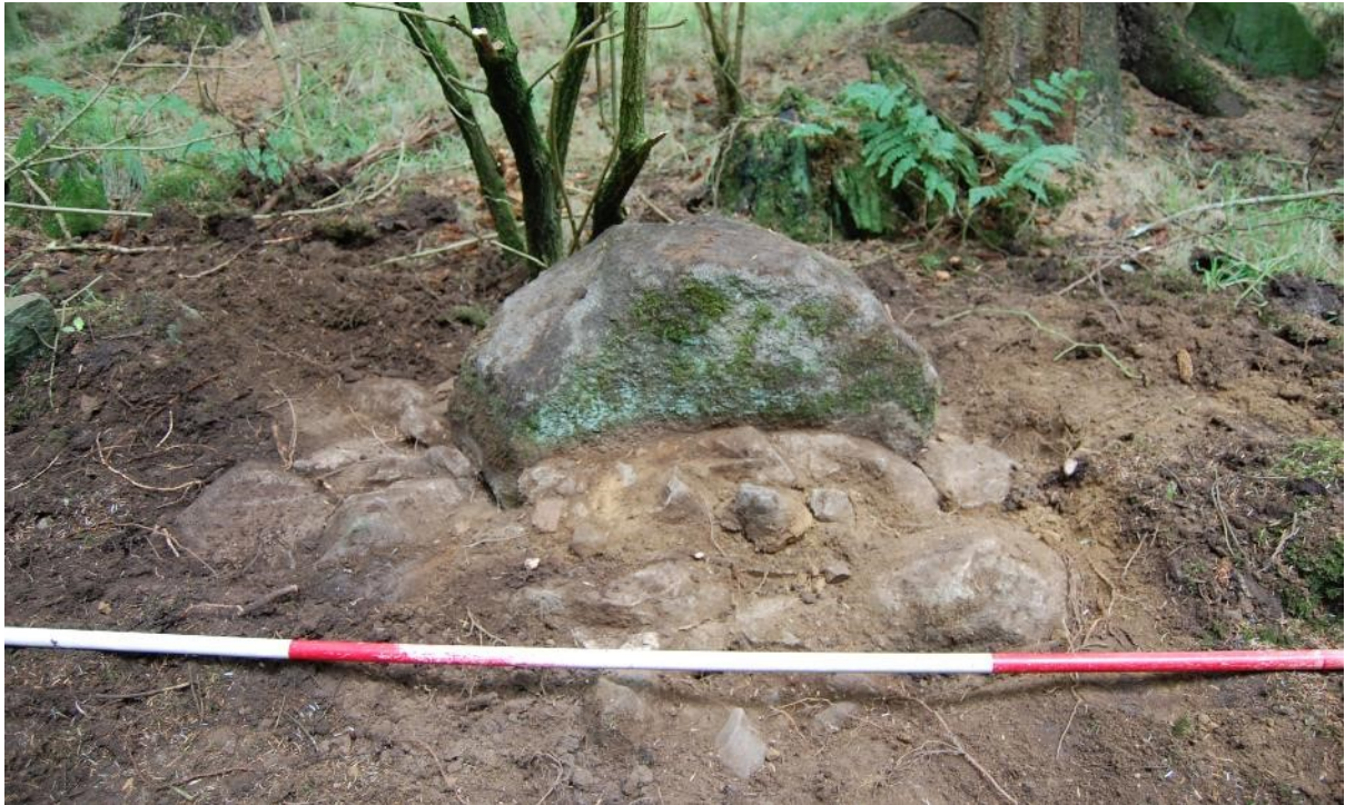
Illus 40 S wall foundation with large curved stone left and reused in Phase 3; facing S
