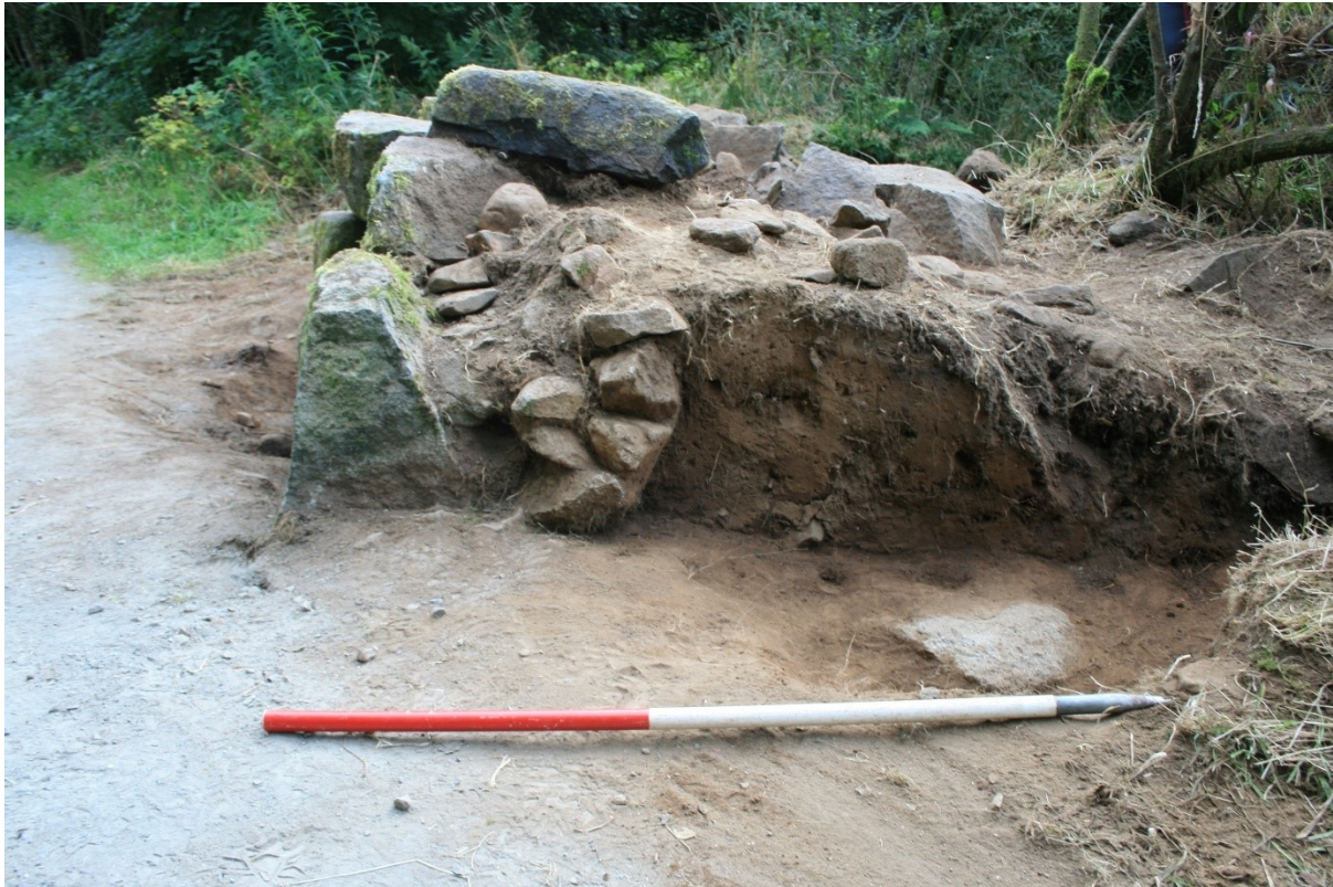
Illus 81 539 S façade showing soil infill behind steps and no evidence of steps on S side of wall; facing N
