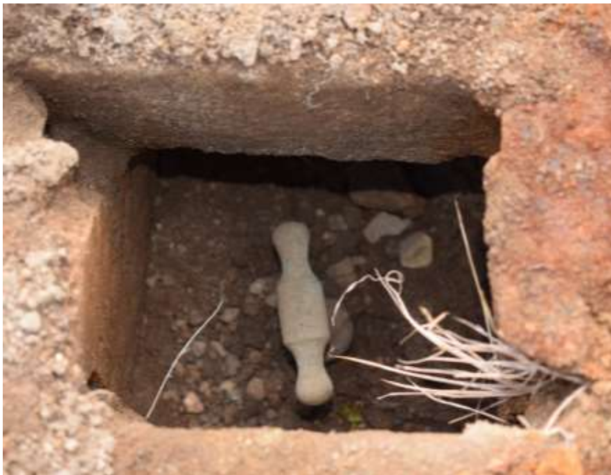
Illus 17 Cast iron hatch 108 with copper tap at base for regulating water to the pond 110; facing E
