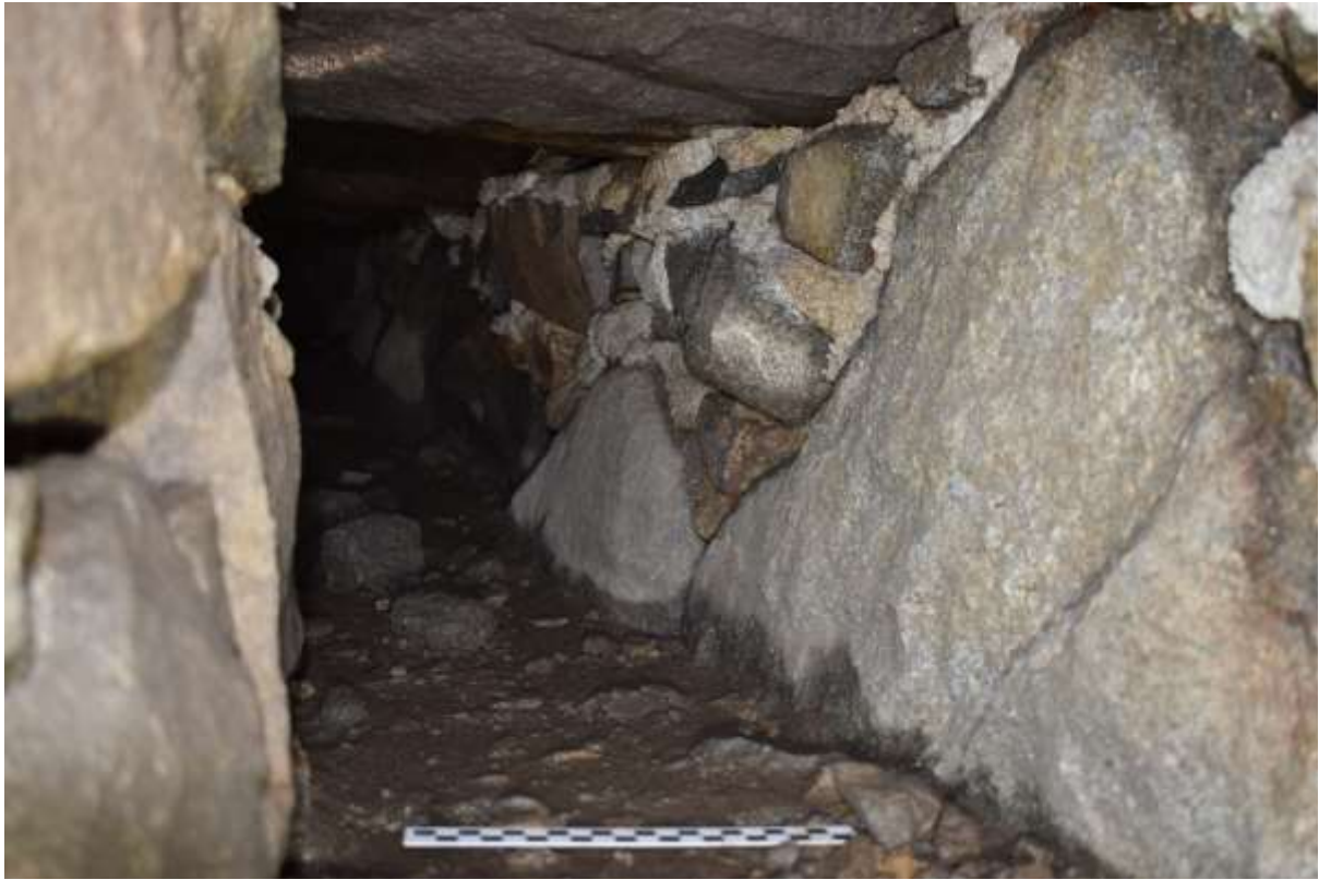
Illus 29 Trench 11 drain 1109 E wall mortared into Mansion W wall foundation
