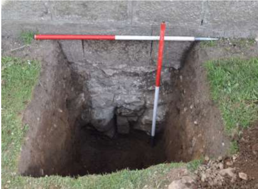
Illus 31 Trench 12 showing foundation of Mansion 0.6m deep; facing E
