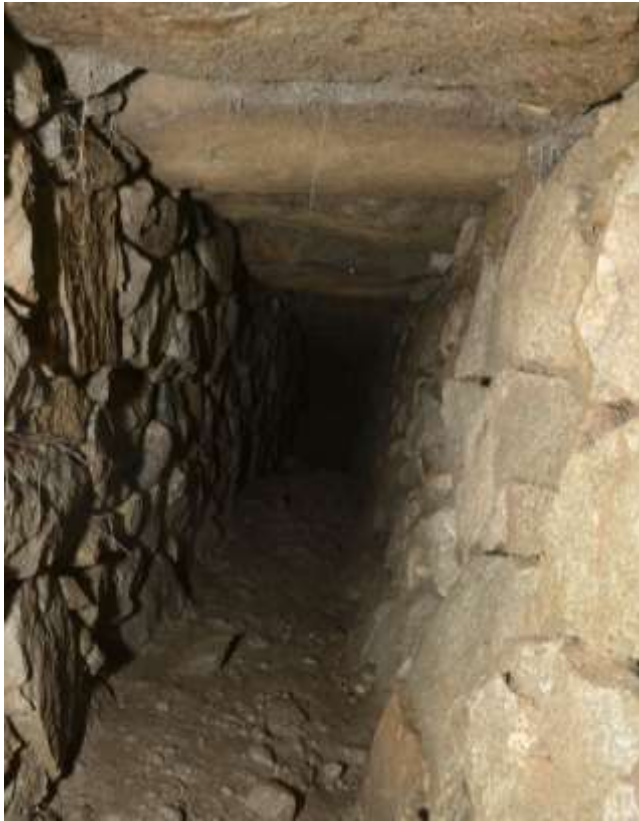
Illus 12 Drain 122 facing W (thanks to Jamie Cutts, Aberdeenshire Council)
