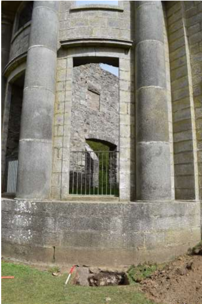
Illus 24 Trench 10 location under ashlar bay window; facing NE
