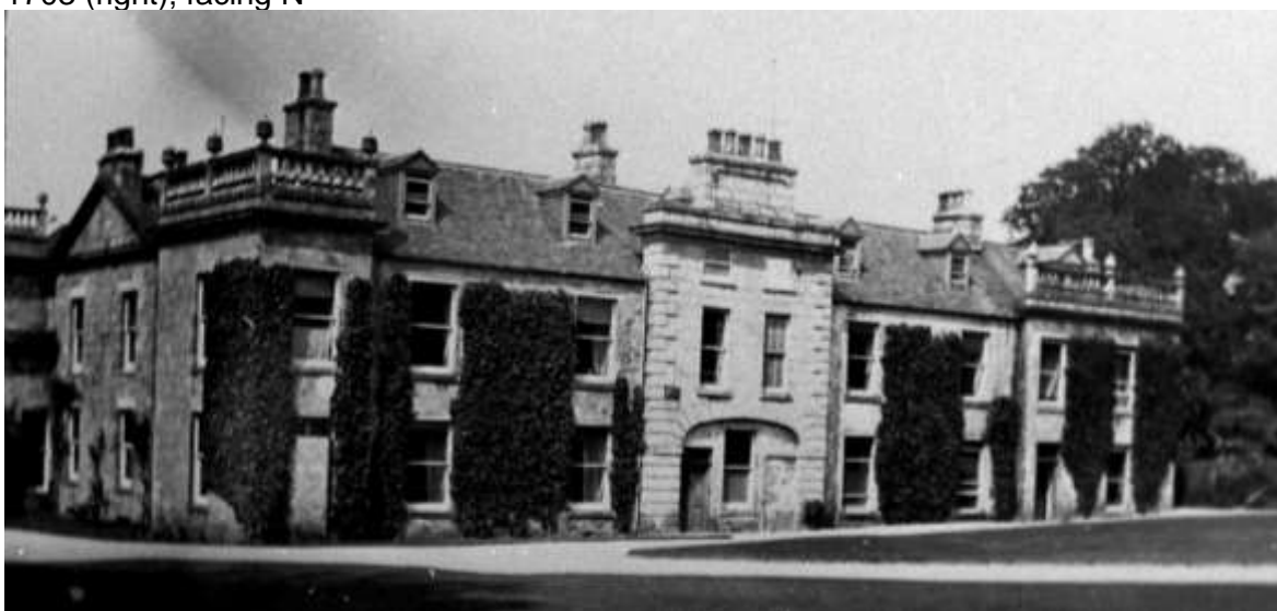
Illus 38 Cart door (centre) showing infilling with stone and brick wall (1703); facing NE (copyright Aberdeenshire Council)
