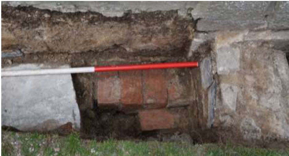
Illus 37 Trench 17 concrete floor 1702 (left) bricks underneath and stone wall foundation 1703 (right); facing N
