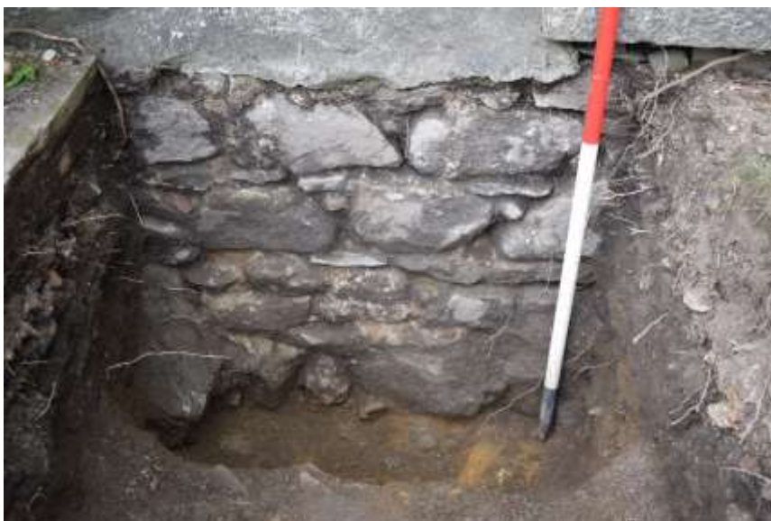
Illus 32 Trench 13 0.6m deep wall foundation under mid 18 th -century Mansion wall; facing W
