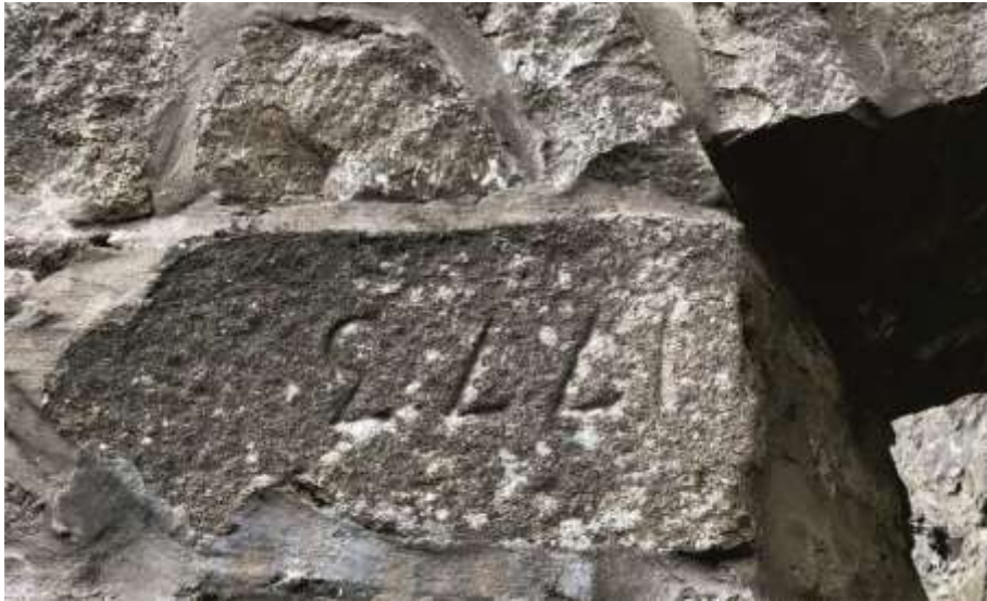
Illus 2 1773 incised date stone reused upside down as the springer for an arch; facing W
