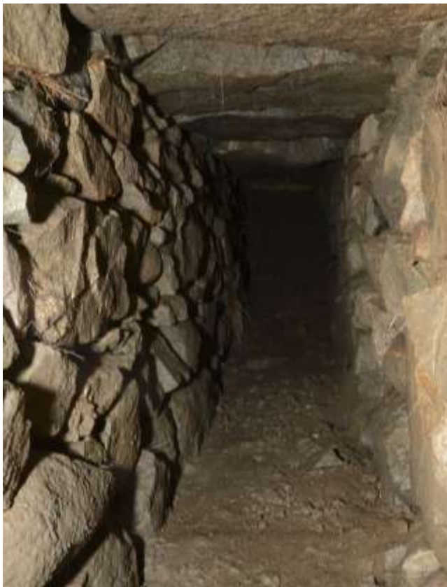
Illus 13 Drain 122 facing E (thanks to Jamie Cutts, Aberdeenshire Council)
