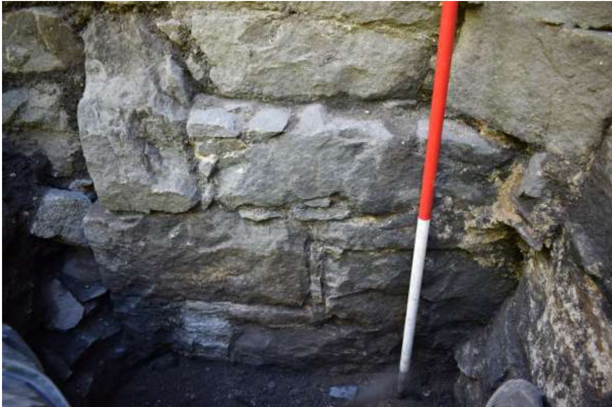
Illus 23 Trench 6 wall 610 (bottom right); not the stone top right is angled at 45 degrees to the current building and features AR/EI incised stone above; facing S
