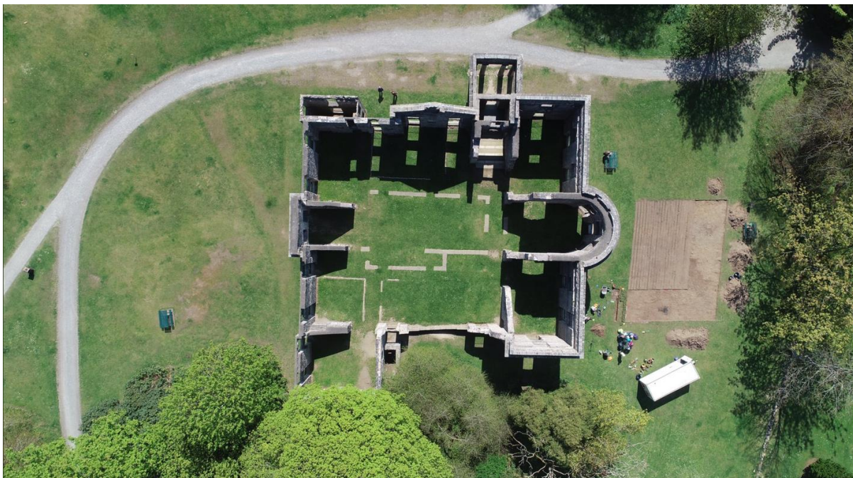
The top elevation helps to illustrate the internal and external layout of rooms and features
