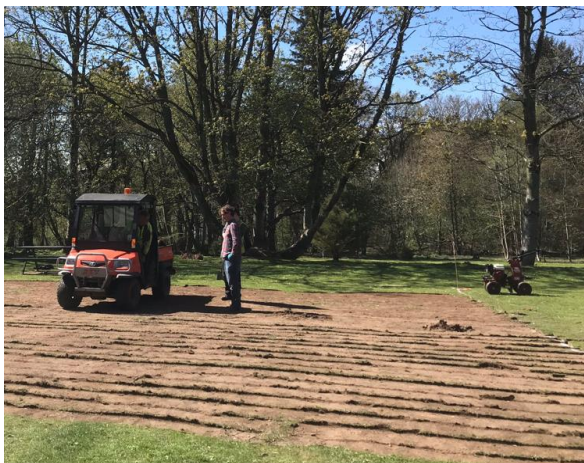
Turf removed from biggest trench
