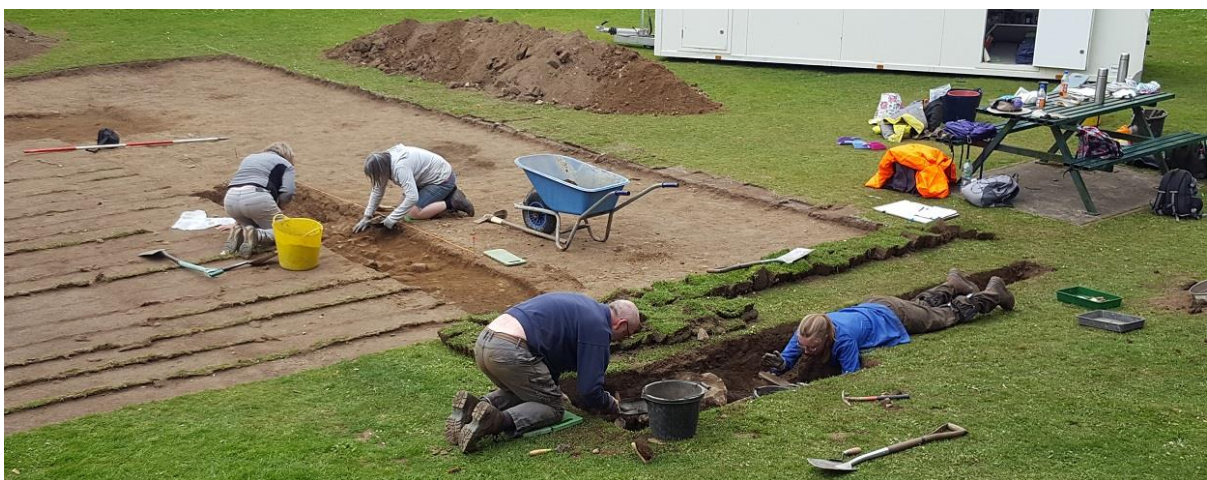
Work continues at what is believed to be a tunnel or drain from the Mansion House
