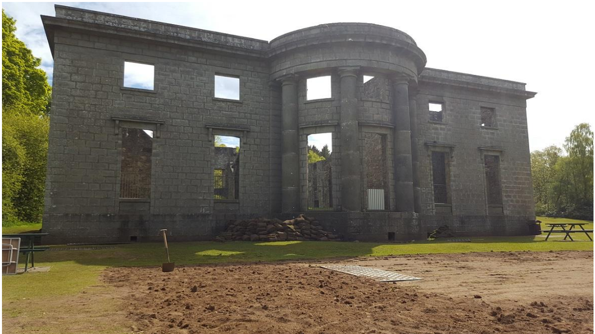
The big trench backfilled
