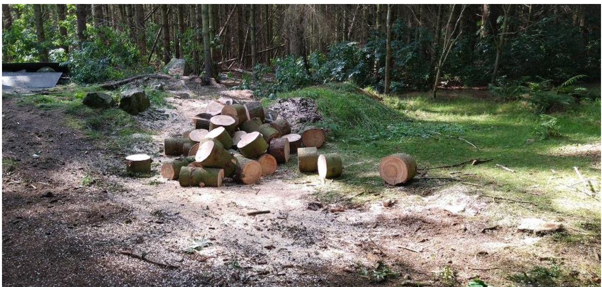
Clearing and removal of the tree on Site 3
