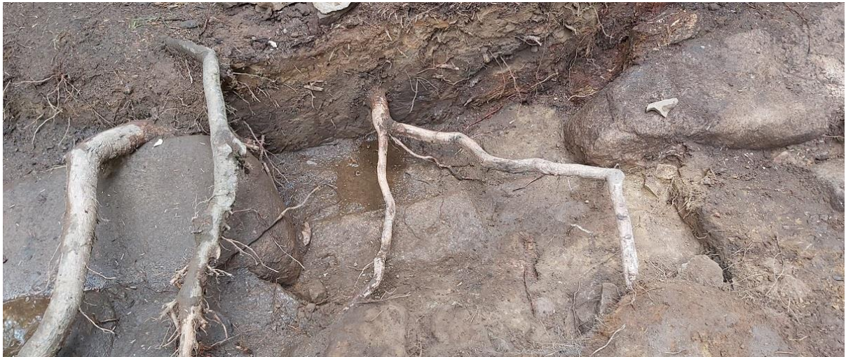
South door cleaned up nicely. Shame about those pesky roots!
