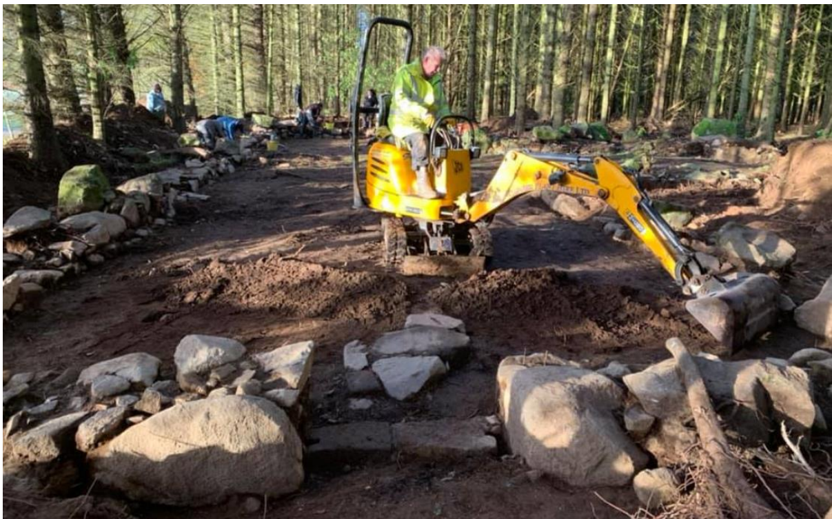
Robbie Cadger starts carefully working on leveling the building interior
