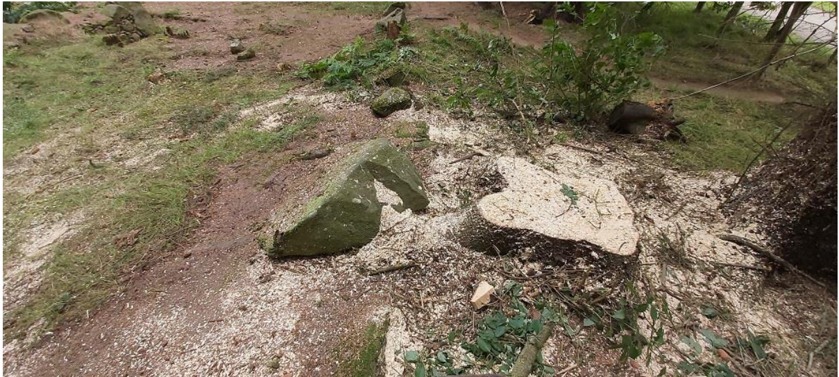
Large tree removed from Site 3 T Shaped Building
