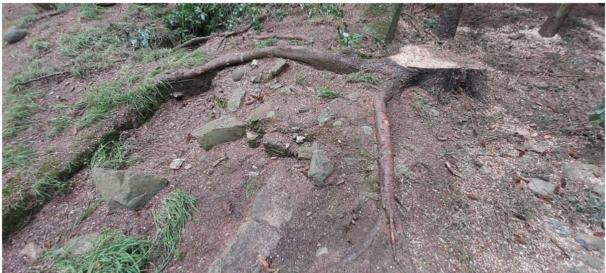
Photographs showing tree removal and remaining roots
