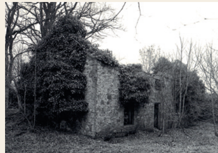
Derelict laundry building prior to renovation
