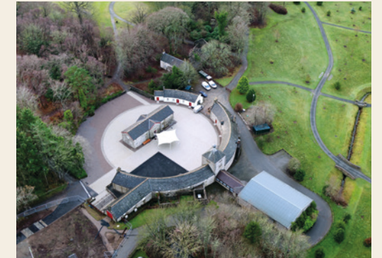
Drone image of the central courtyard
